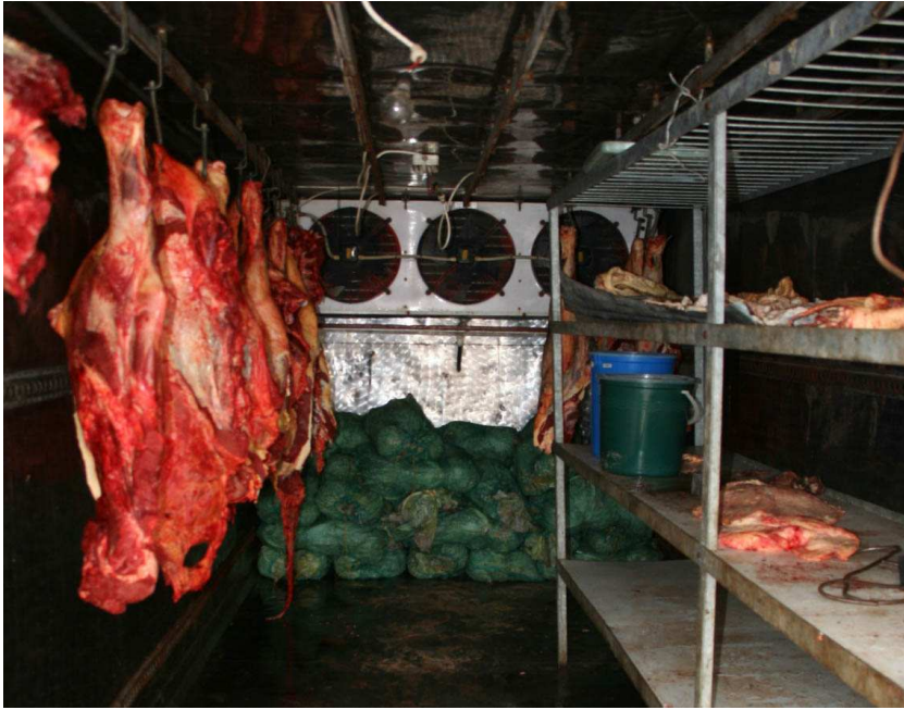
Illustration 8: Typical cold storage facility
